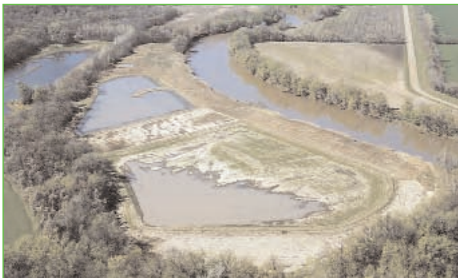
The top photo shows riverbottom farm land prone to flooding and erosion. The bottom photos shows work done after the land was entered into the WRP program. The riverbank will be stabilized, and permanent wetlands that will attract migrating waterfowl, as well as provide valuable habitat for other wildlife, will be created.
